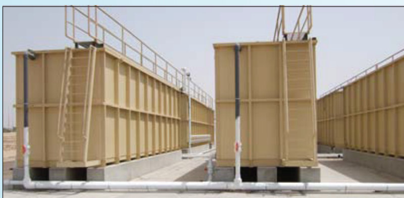
EfloSAF for International City, Dubai. 1000 m 3 /d. TSE < 10 mg/l BOD, SS < 10 mg/l, HN 3 -N < 5 mg/l
